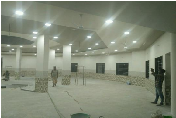
Bhoopali Mess under Construction
